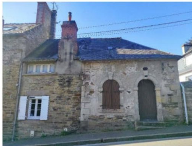
Pavillon, rue Kervenno © BE-AUA
